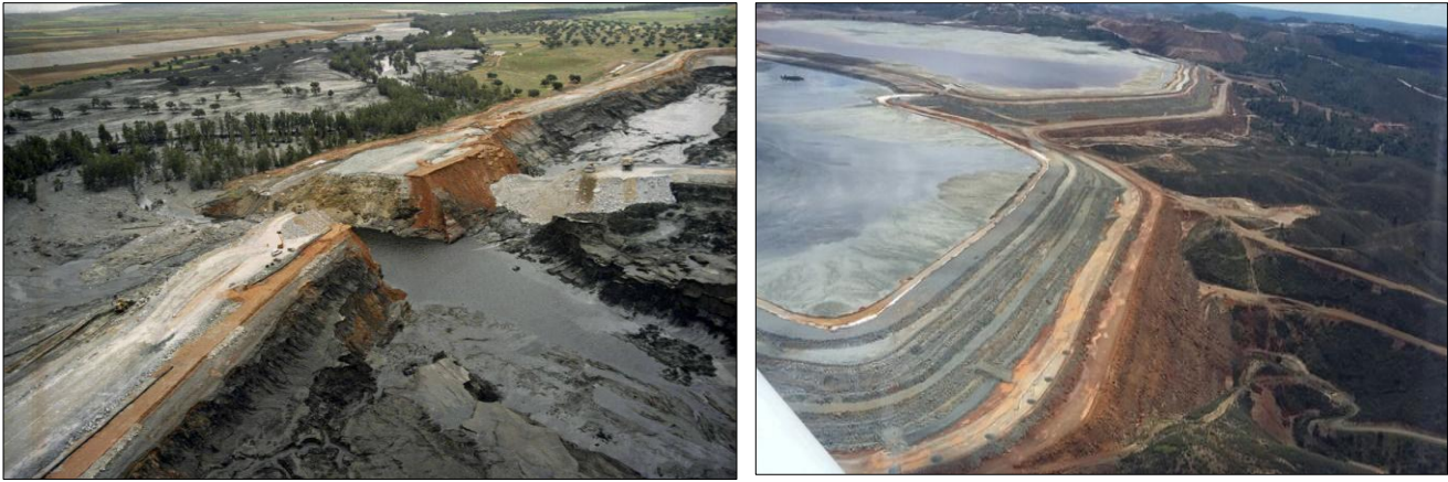
Figure 5 – Aznalcóllar Disaster of 1998
