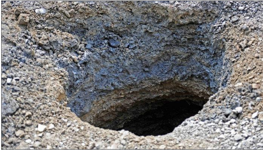
Figure 7 – Deep hole over the old shaft
